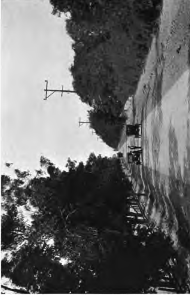
Contra Costa County builds 18 foot roads and the clearance supplied is well shown in this picture.
